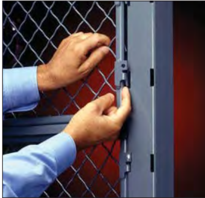
STEP 1: ALIGN HOOKS AND INSERT INTO SLOTS
